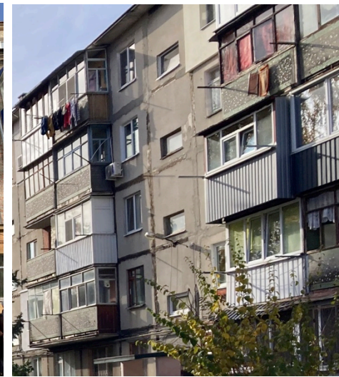
Increase in living space by extending and glazing balconies with a ledge
