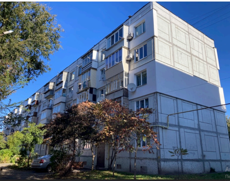
Individual implementation of measures for facade insulation, as well as the installation of air conditioners and satellite dishes to enhance the comfort and functionality of housing
