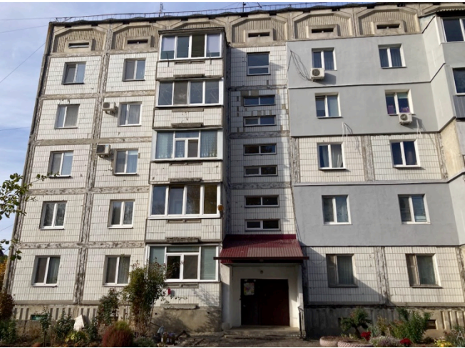
Individual implementation of measures for facade insulation, as well as the installation of air conditioners and satellite dishes to enhance the comfort and functionality of housing
