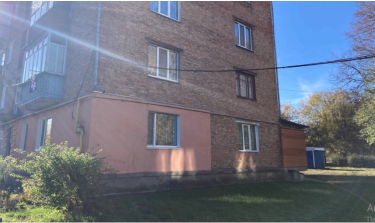
Increase in living space by extending and glazing balconies with a ledge
